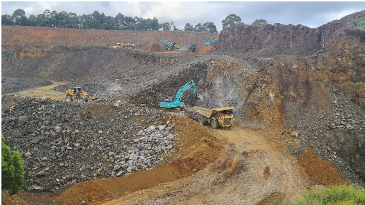
Figure 1 - Image of the new “Land bridge” in operation, November 2022
