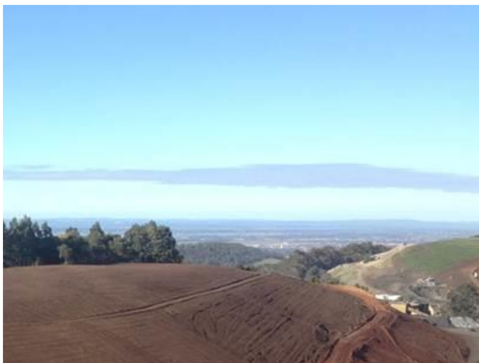
Figure 2: Part of the extraction area to be rehabilitated after topsoil was spread over the site.
